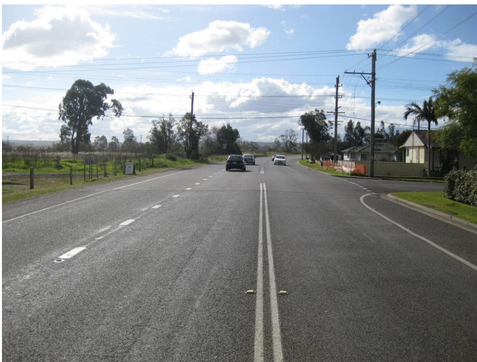
View looking north along TC Frith Avenue at Second Street.
